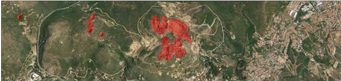
Eroded areas due to excavations over Monteponi
