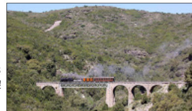
infrastructures complementary railways of Sardinia
